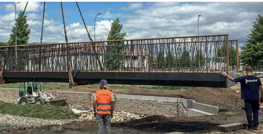
Installation on location of a prefab bridge in Châlon-Sur-Saone, FR
