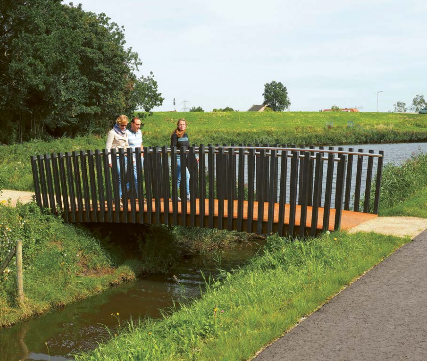
In this sustainable Solo Bridge the entire carrier and deck construction are made of thick-walled CorTen steel plates. The posts of the fence are of Solid All Black composite beams. Meanwhile the warm brown deck is provided with an anti-slip pattern using the same CorTen plate.
