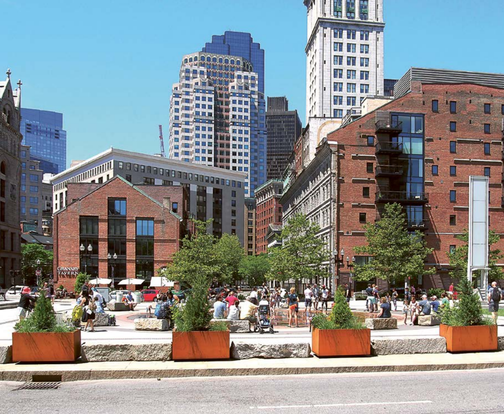
These days, increasingly strict requirements are applied to protect strategic (government) buildings and public spaces. The complete safe shielding of buildings, preventing ram raids and attacks, is considered high priority. In this Boston square, Shrubtubs Square are interspersed with granite blocks. The designers have succeeded in creating an unobtrusive barrier.
