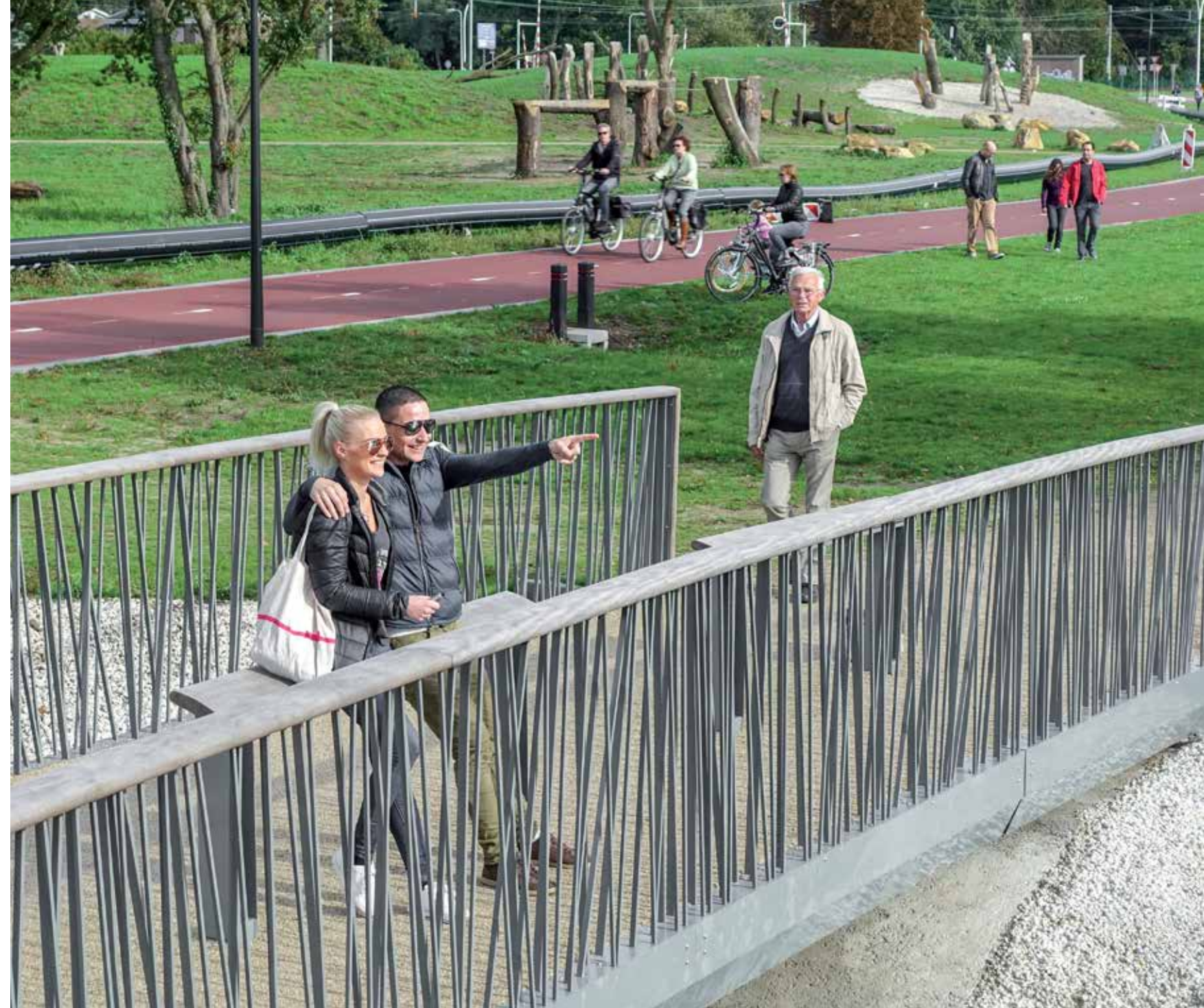
This 12-metre-long coated Bowie bridge was installed in the Watertorenpark in Hengelo, the Netherlands. The 3-meter-wide bridge has standing seats in the middle, inviting passers-by to stop for a moment and enjoy the view of the park.
