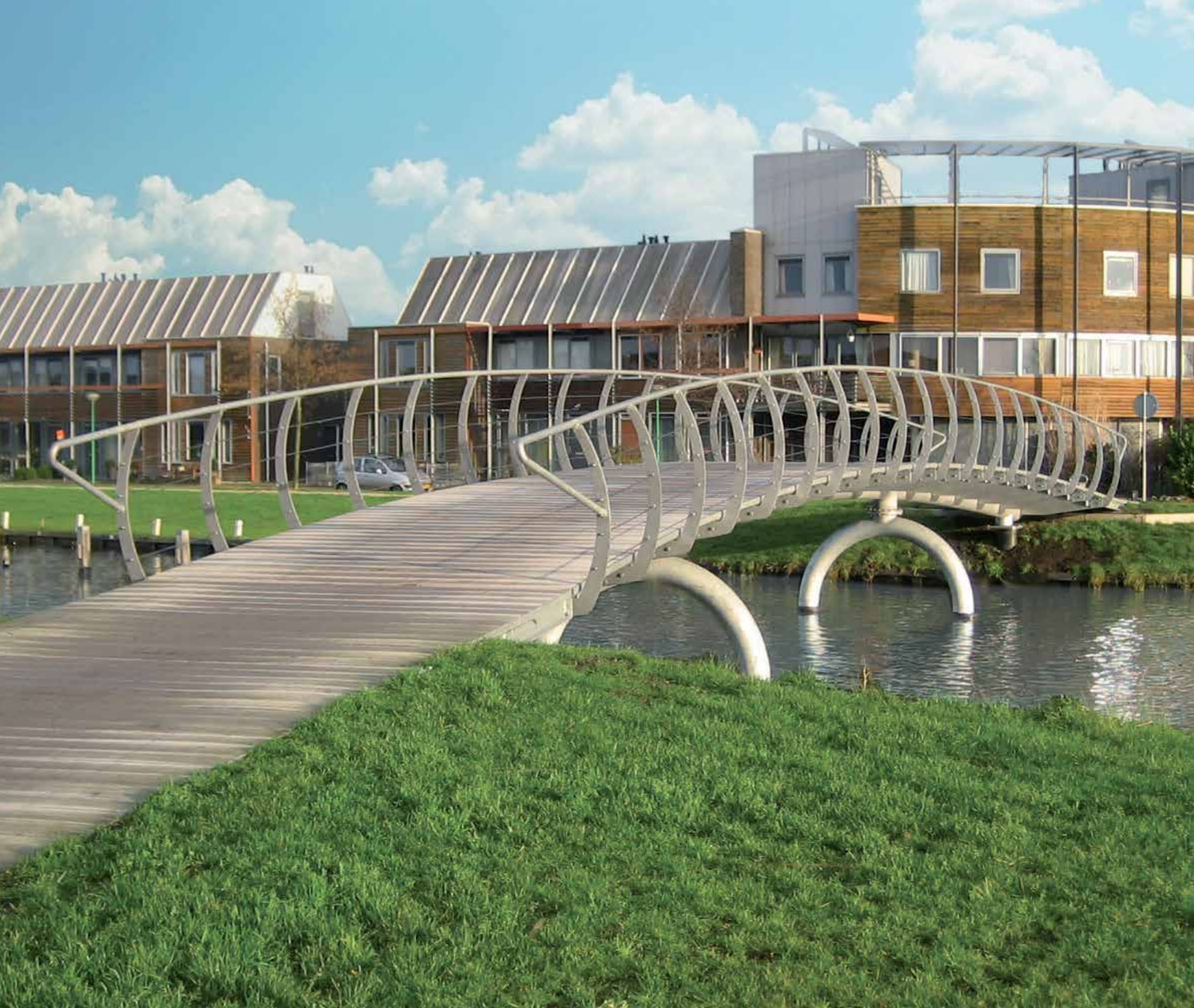
This 30-metre-plus long striking Inline Bridge has been placed in a new residential area in Sneek (NL). The two supports have been installed from the bank. The many boats that pass under the bridge were accounted for by designing a spacious passage.
